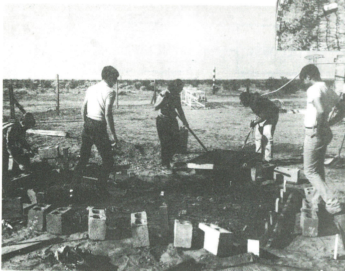
The first load of cement is readied for the blockhouse
