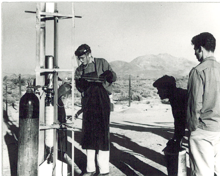
Photo 11 - Lee Rosenthal adds 90% hydrogen peroxide to the propellant tank just prior to the flight. The auxiliary nitrogen tank has been connected to pressurize the flight nitrogen tank. Part of the aluminum shell can be seen resting on a crosspiece in the tower just above the rocket.
