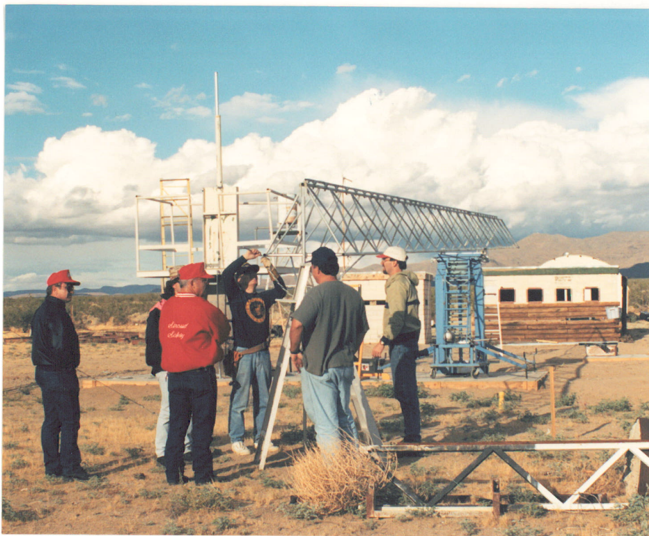
The assembled tower is mounted on the hydraulic man-lifter just prior to raising.
