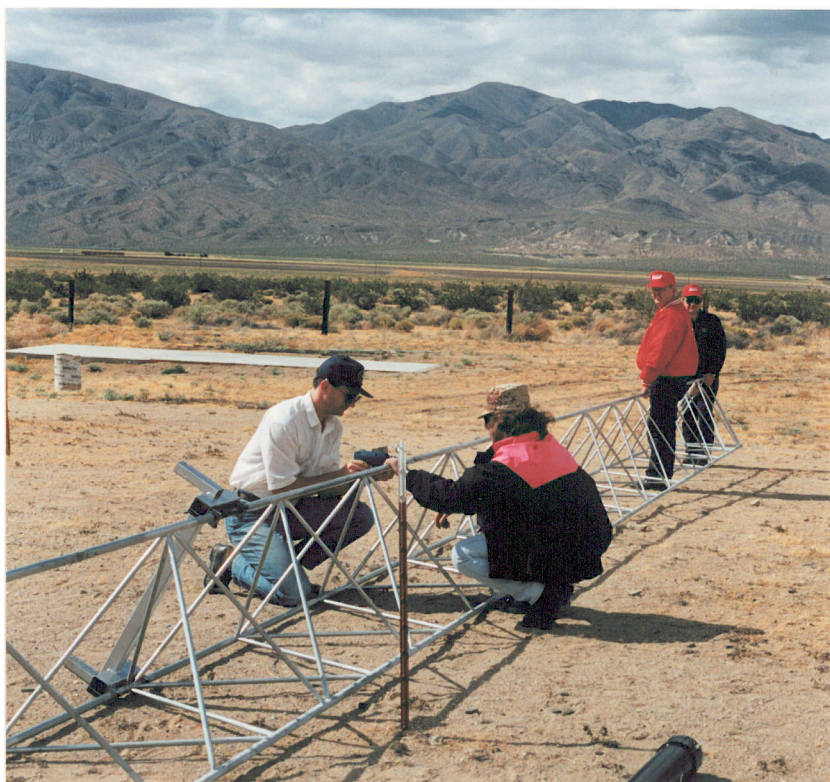
The start of the tower assembly. The six, ten-foot long sections are being bolted together prior to installing the launch rail.
