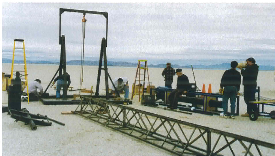
Assembly of the launch tower from all its component parts is a few hour job for utilizing all available hands.
