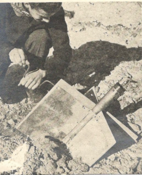
At its destination spent rocket is dug from salty earth in which it buried itself on landing. Tail is then removed for easier handling, and a brace is used to take covers off fins.
